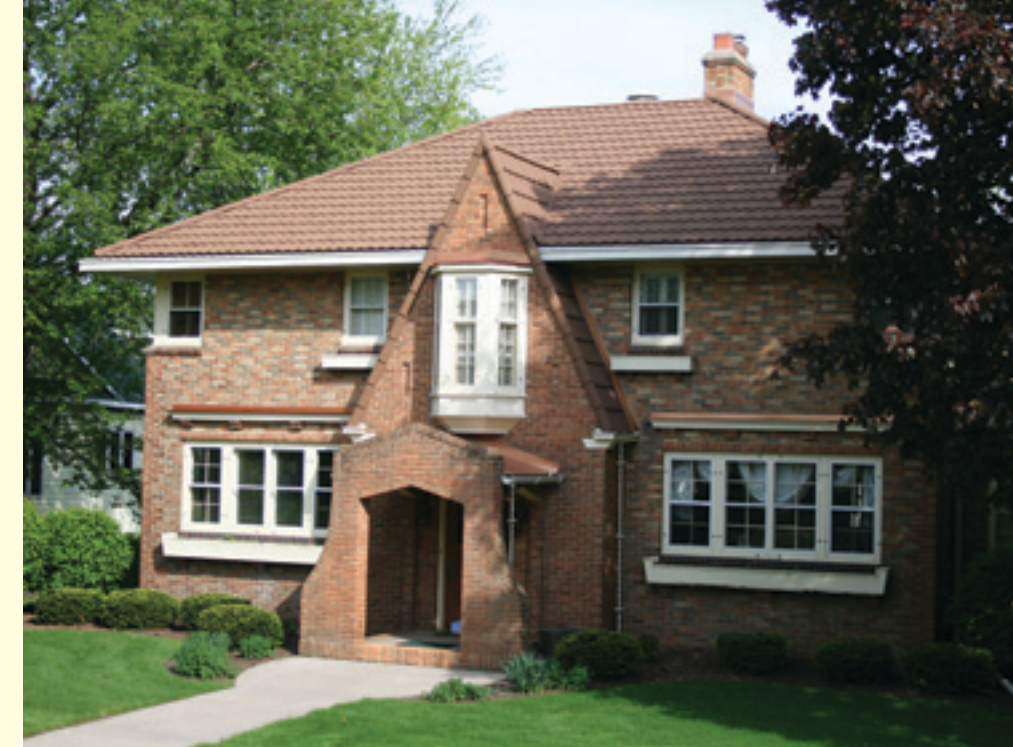
This DECRA roof still looks great after the recent hailstorm.
